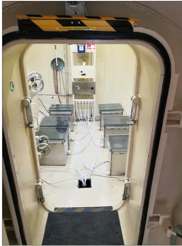
Figure 1. Semi-hermetic monoplace boxes placed in the hyperbaric oxygen chamber and their connection to the oxygen system.
